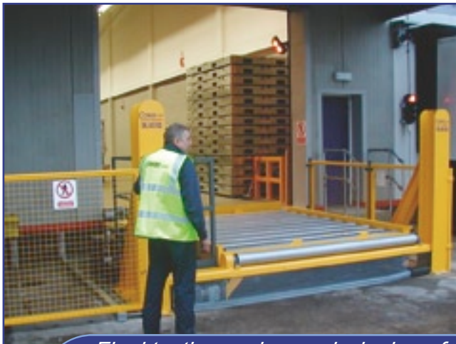
Final testing and commissioning of equipment prior to handover.
