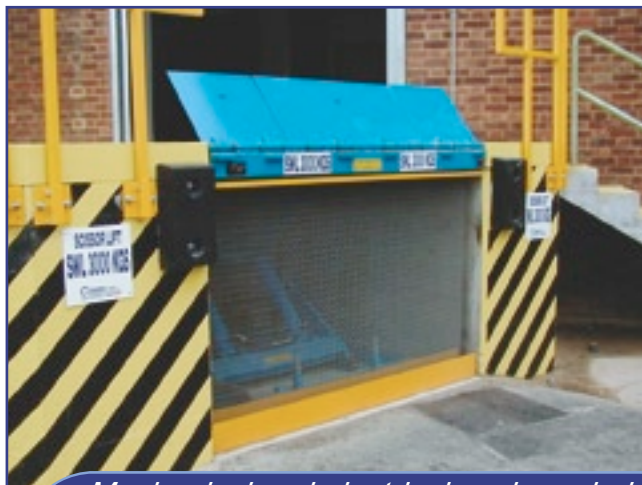
Mechanical and electrical work carried out by our own expert installers
