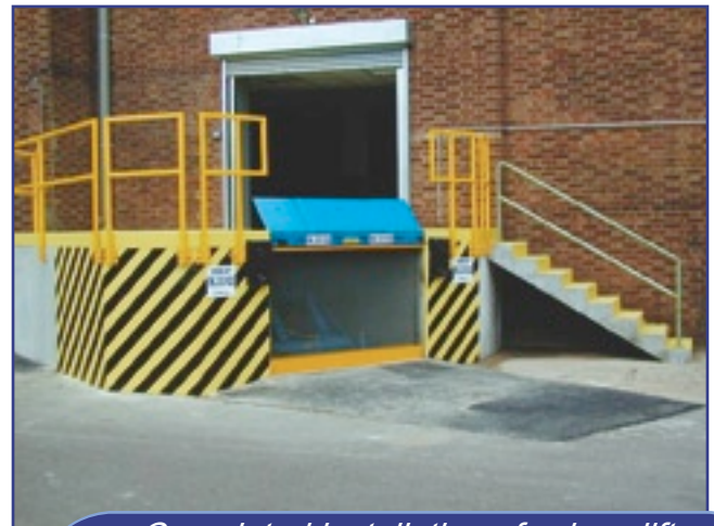
Completed installation of scissorlift equipment in less than 3 days.
