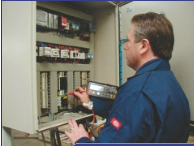
Air Conditioning Systems
